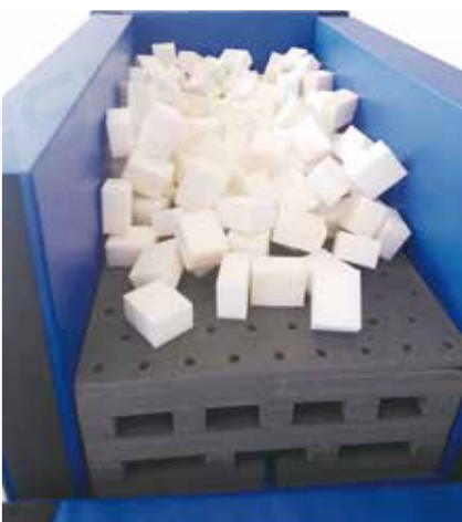
Bottom structure of the foam pit
